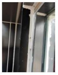
Figure 8: 8mm hole at 3/4 window height in caulking
