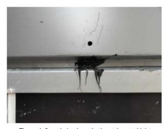
Figure 4: 8mm hole above horizontal control joint
