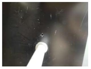
Figure 7: 8mm hole above pipe penetration
