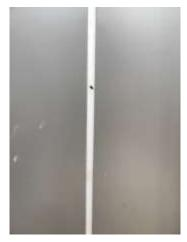
Figure 6: 8mm hole in panel joint caulking
